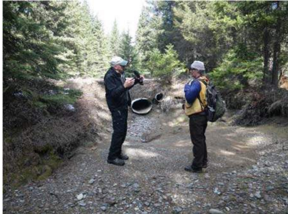
Figure 39. Undersized culvert.
