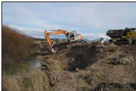
Figure 32. Floodplain excavation on the Reimer reach.
