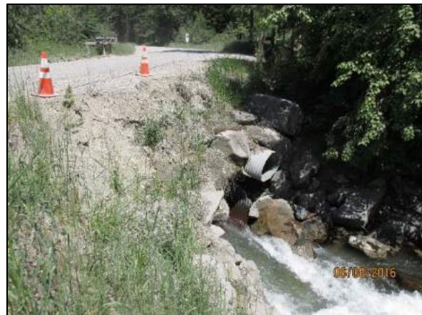
Figure 35. Downstream end of Haskill Basin Rd. culvert.
