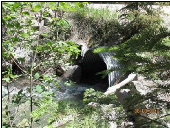
Figure 34. Upstream end of Haskill Basin Rd. culvert.
