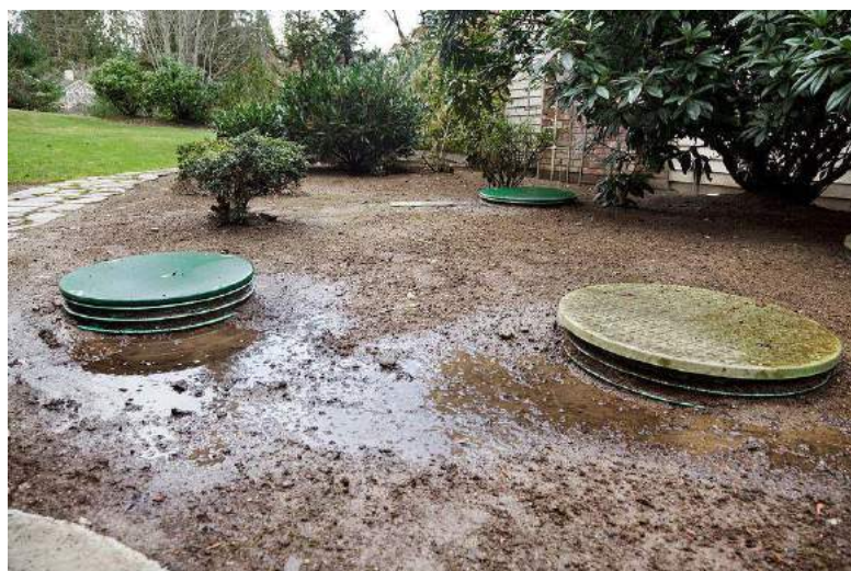
Figure 14. Leaking septic system in a residential yard. Surface leaks such as this can runoff over surfaces and impair nearby waterbodies ( www.hardwareandtools.com ).
